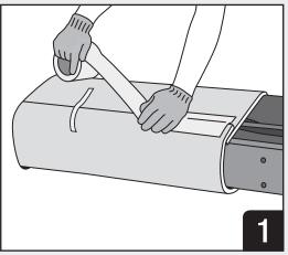
At the opening, install 3M<sup>™</sup> Interam<sup>™</sup> Endothermic Mat E-5A-4 in a single width mat around the protected item, tightly butted up to the opening. Overlap the cut edge a minimum of 50mm. Close all cut edges with 3M<sup>™</sup> Aluminum Foil Tape 425. E-Mat may be temporarily retained with 19mm wide filament tape.
