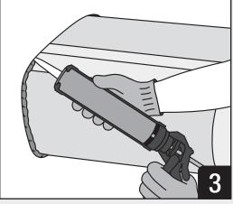
Fill any gaps to the depth of the E-Mat with 3M<sup>™</sup> Fire Barrier Sealant CP 25WB+ or 3M<sup>™</sup> Fire Barrier Water Tight Sealant 3000 WT Sealant. Fill annular space in any through-penetration scenario as per system specifications. Close all filled gaps, joints between sections, and overlapping sections with 3M<sup>™</sup> Aluminum Foil Tape.
